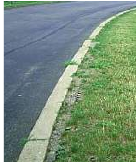
Asphalt road with flush concrete kerb
