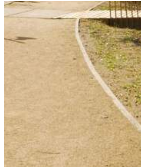
Compacted granitic gravel path
