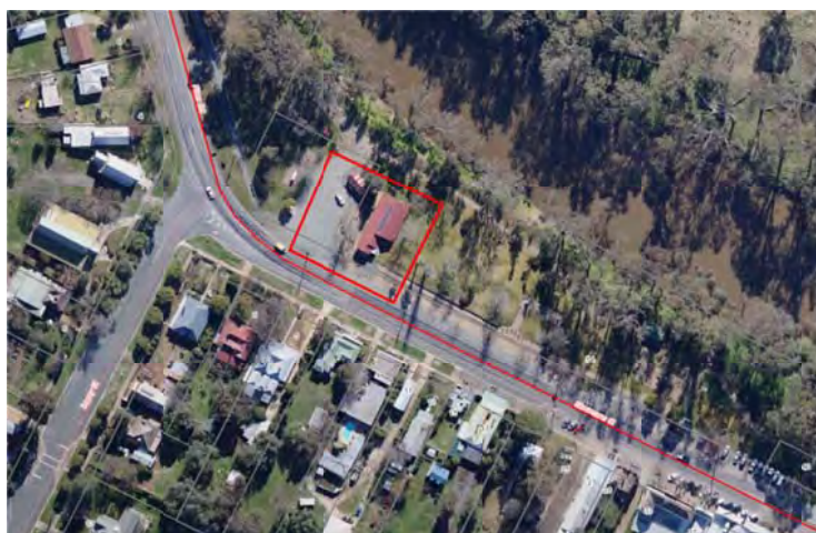
Murchison Heritage Centre Stevenson St Murchison VIC 3610
