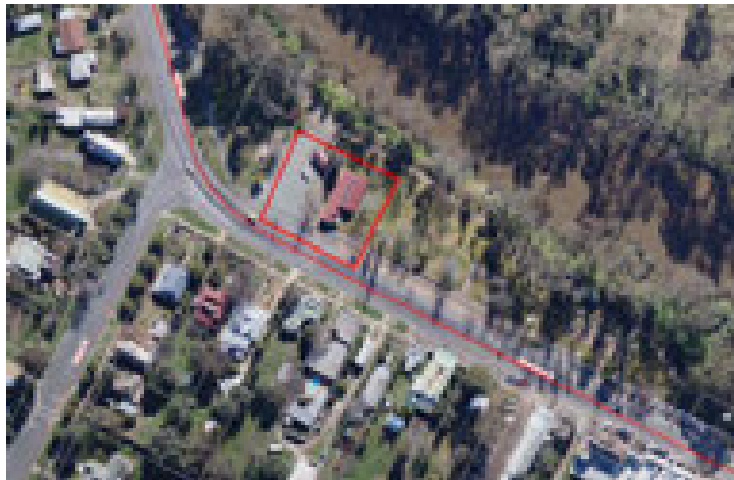
Murchison Heritage Centre Stevenson St Murchison VIC 3610
