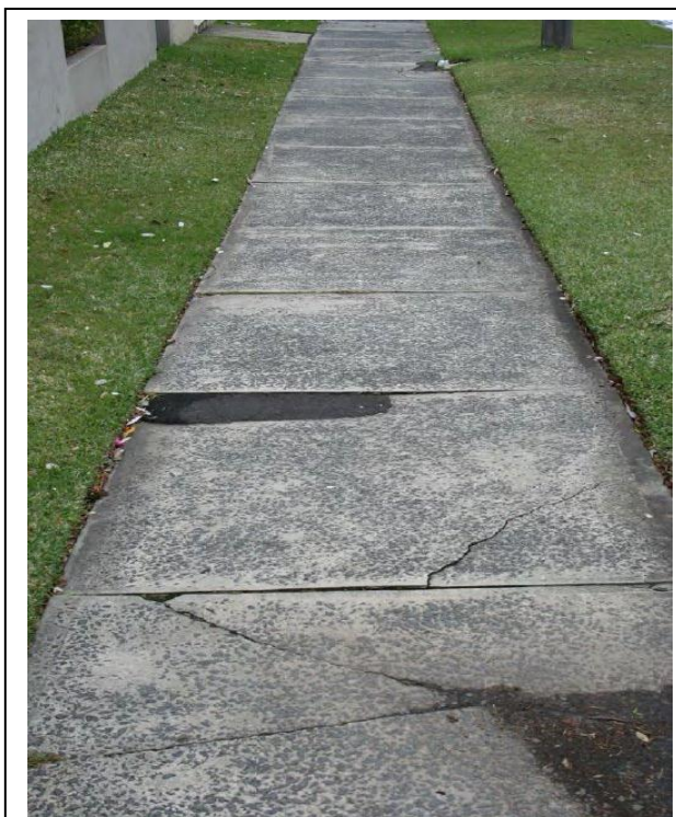
Footpath in fair condition (5 to 6 rating)
