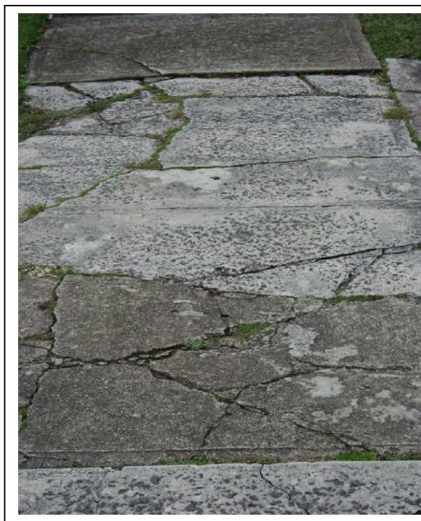
Footpath in poor condition (8 to 9 rating)
