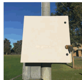
Irrigation cabinet example
