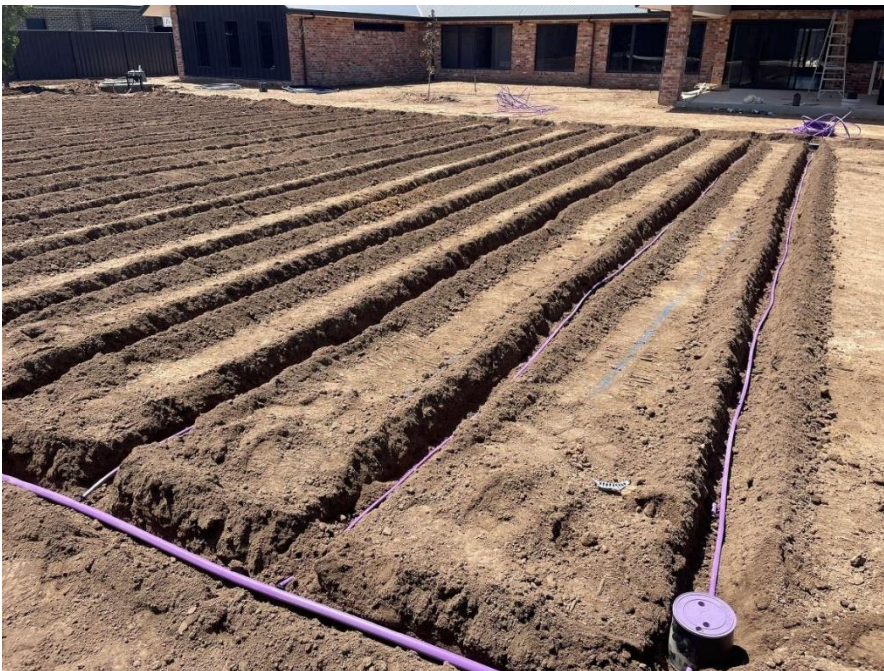
Image 19: pressurized sub-surface drip irrigation
