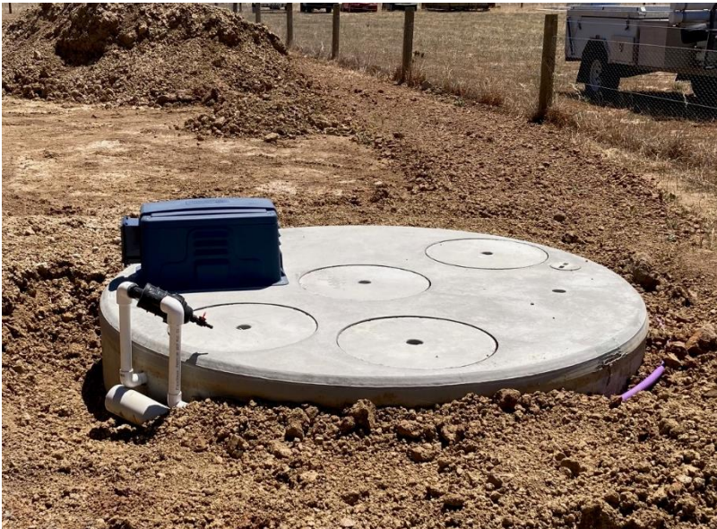
Image 10: Top of a packaged treatment plant – only the lid, control box and filter visible once backfilled
