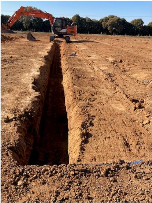
Image 17: Excavation for a Wick Trench
