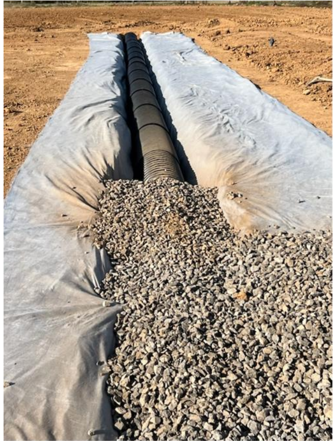
Image 18: Backfilling of Wick Trenches, with Geotextile fabric lining the trench before backfilling with suitable sized rock and arch drain.
