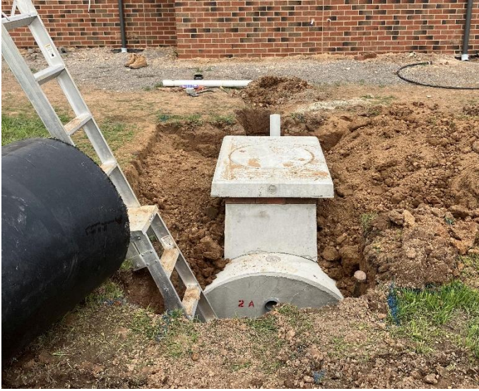
Image 9: Only the lid of the septic tank and pumpwell with alarm are visible when backfilled.
