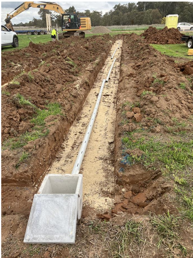
Image 12: Evapotranspiration trench with gypsum sprinkled along the bottom of the trench. Trench is 400mm deep and 1m wide
