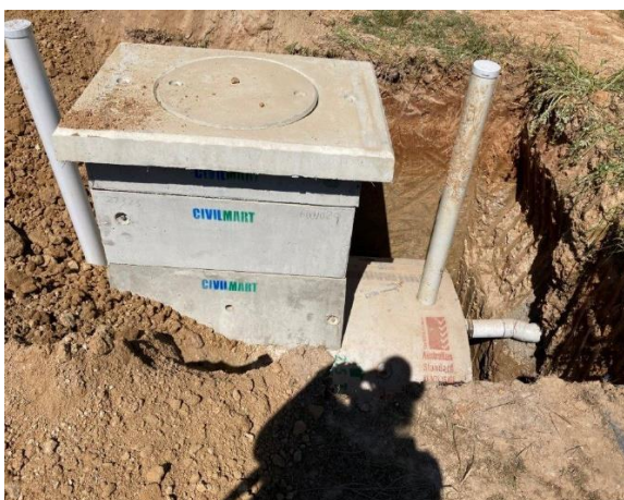
Image 8 – Septic tank with riser lids finished at ground level. All waste septic tank with risers extended to ground level to ensure access for pump out and other maintenance. Pump well installed at the outlet of the septic tank to pump to effluent disposal trenches.
