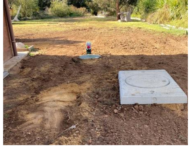
Image 9: Only the lid of the septic tank and pumpwell with alarm are visible when backfilled.
