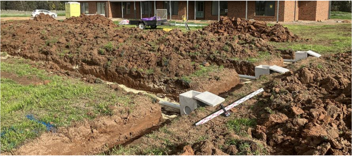
Image 15: An example of trenches laid in a series, spaced 2m apart.
