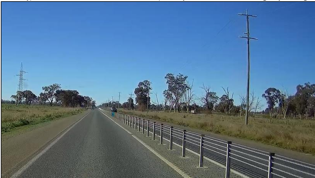
Photo 2: Typical cross-section of the centreline wire rope safety barrier on the Midland Highway, looking east
