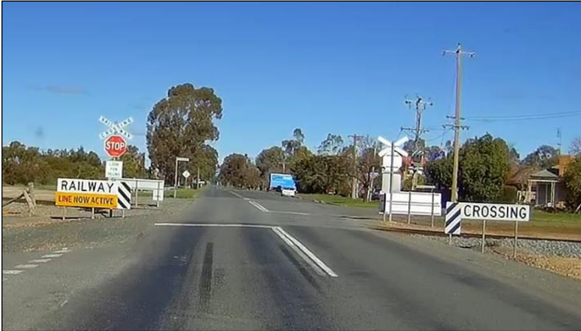
Photo 16: Dhurringile Road rail crossing
