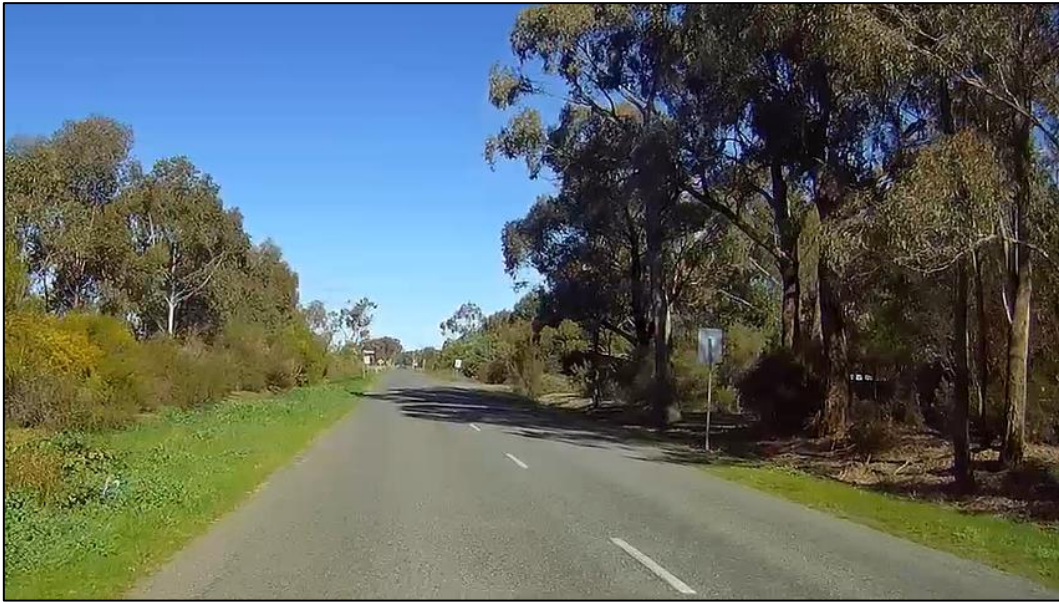
Photo 12: typical rural residential cross-section of Dhurringile Road, looking north
