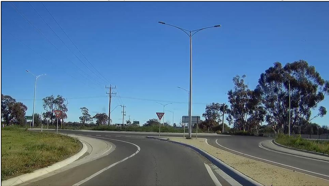
Photo 1: The Midland Highway intersection with the Tatura-Undera Road, looking west
