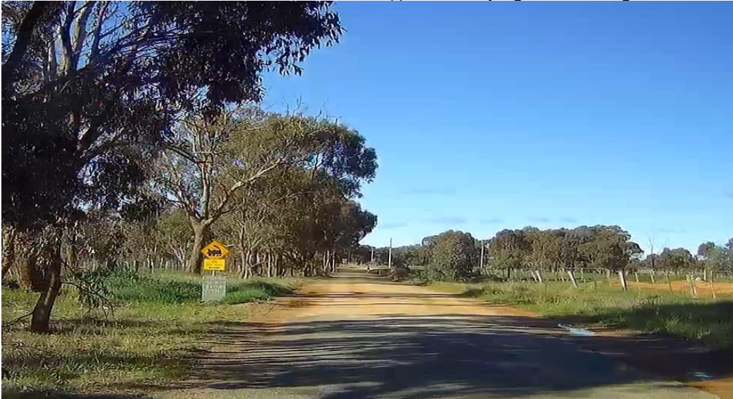
Photo 10: Cross-section of Murton Road on approach to Bayunga Road, looking east
