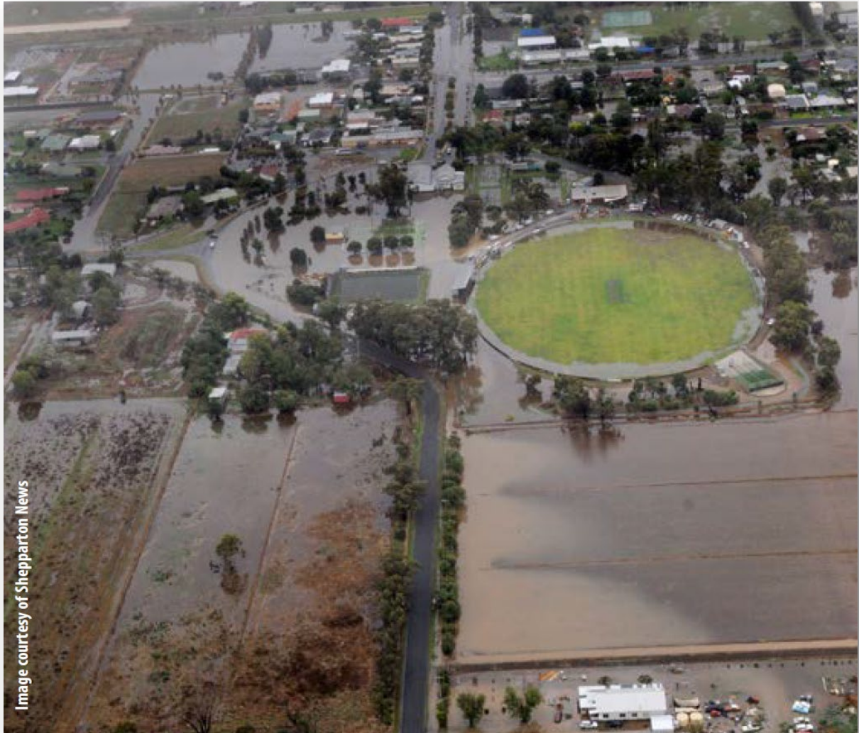
Aerial view of flooding at Katandra West in March 2012 (source: Katandra West Local Flood Guide, December 2016)
