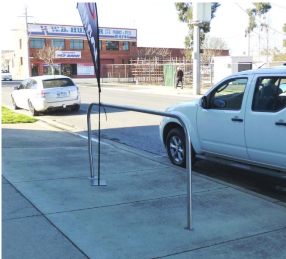
Figure 6.10: Bicycle Parking Hanging Rail
