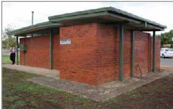
Facility is not clearly signed with no defined access
