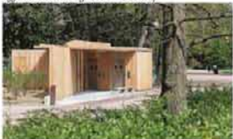
Public toilet in parklands support an active lifestyle in a community. http://openbuildings.com/buildings/public-toilets-in-the-tote-dor-park-profile-44712
