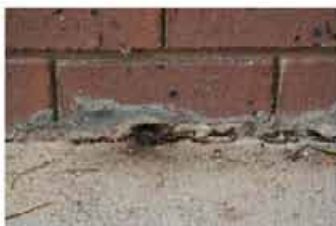
Building floor does not drain effectively. Holes have been drilled into wall to help water drain out. Jaycee Park, Murchison.
