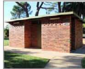
Free standing brick facility
