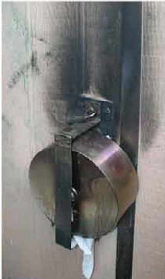
Toilet roll dispenser which has been set on fire Ducat Reserve, Shepparton
