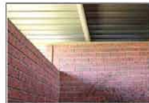
Poor internal natural light minimal and evidence of graffiti
