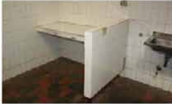
Change table at the Water Tower Gardens facilities is in poor condition and unsafe
