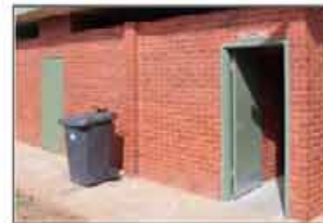
Entrances to cubicles are not inviting
