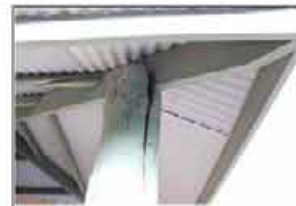
Split timber purlins requiring repair/replacement
