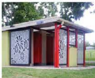
Perforated steel screens. http://www.cocoonedesign.com.au/g-our-workpublic-amenities-refurbishments
