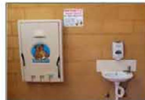
Baby change not adequate for facility
