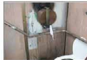
Evidence of vandalism and graffiti
