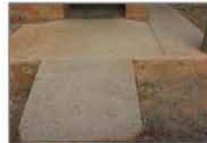
Recent modifications to concrete path
