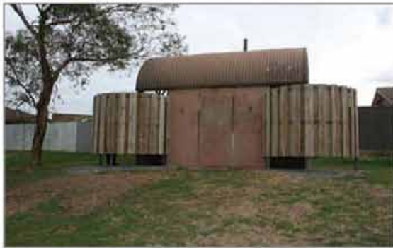
Facility is not accessible, minimal signage, and strong negative perception
