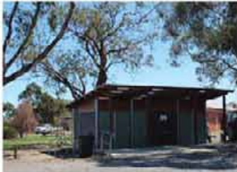
Recently installed public toilet facilities Undera
