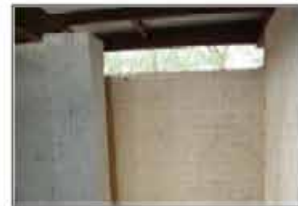
Bugged brick finish walls appear dirty
