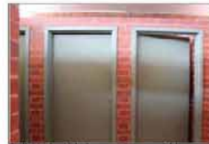
Individual cubicle doors are heavy and fully enclose each cubicle
