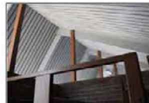
Internal natural lighting not adequate
