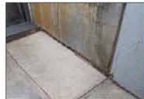
Building in poor condition
