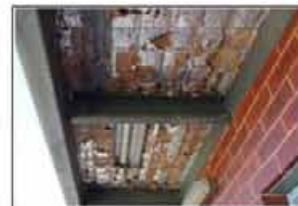
Damage to insulation externally
