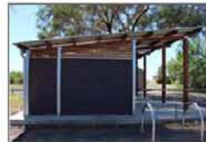
Building design allows natural light into facility
