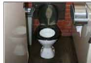
Fixtures and fittings used but generally in good condition
