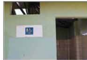
Signage and open entrance
