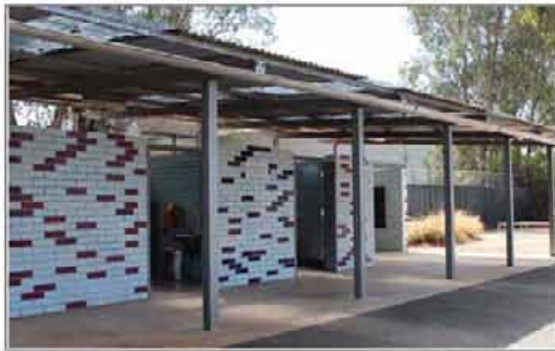
View from within fenced area. Open access and circulation around facility entry
