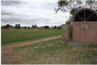
Toilet located in residential area and disused sports field Ducats Reserve, Shepparton
