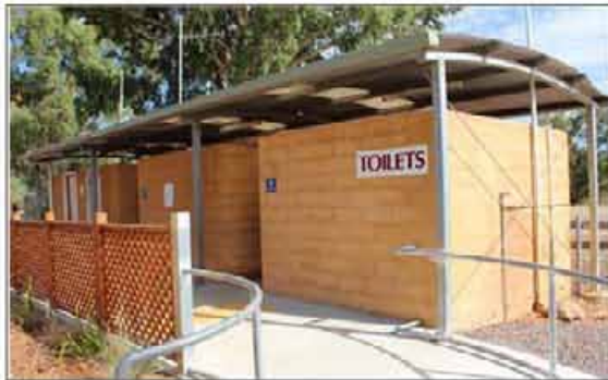
Free standing building within play and community facility
