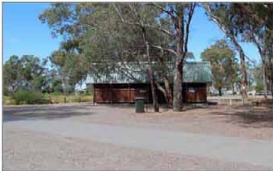
Stand alone building between the lake and camping reserve
