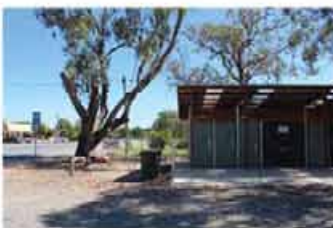
Toilet close to main road Undera
