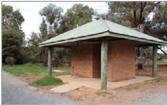
View of facility from the car park. Bushland track to the left with large shrubs obscuring sightlines
