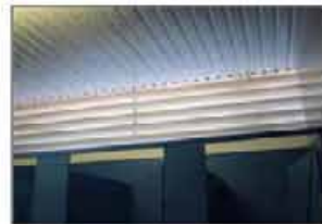
Inadequate internal natural lighting
