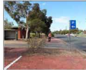
Toilet block obscured from main street
