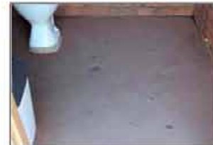
Inadequate turning space in accessible cubicle
