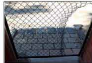
Evidence of vandalism
