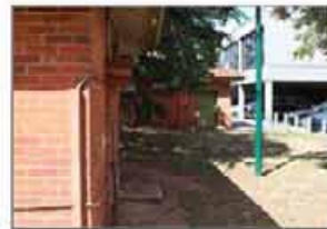
View to rear of buildings obscured
