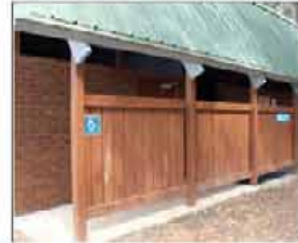
Timber modesty screens to cubicle entrances
