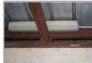
Inadequate, aged lighting
