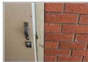
Evidence of vandalism
