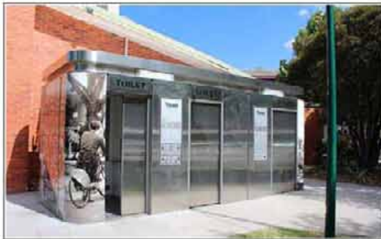
Steel facade with feature graphics and fully automated doors
