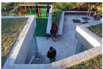
Public toilets close to play and activity areas, such as this one, help increase participation in recreational activity. http://inhabitat.com/green-roofed-public-restroom-facility-in-argentina-offers-amazing-river-views/
