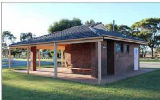
Free standing brick building within cemetery, incorporated into shade structure: waiting area
