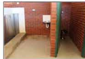
Fixings are aged but well maintained
