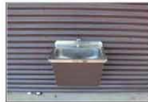
External wash basin
