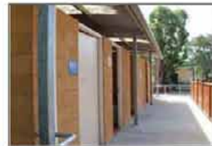
All entrances along traffickable side
