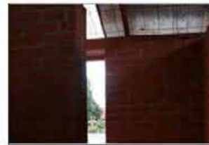
Inadequate internal natural light
