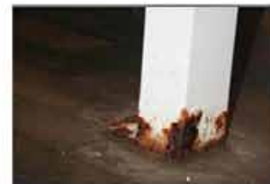
Structural damage to building due to inadequate drainage
