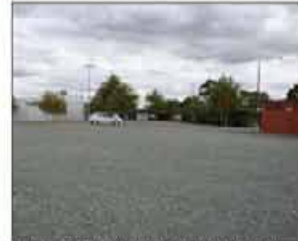
Clear views to building, no defined access with large expanse of asphalt surrounding
