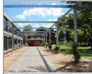
Defined path to male facilities, undercover car park to left, and gardens to right
