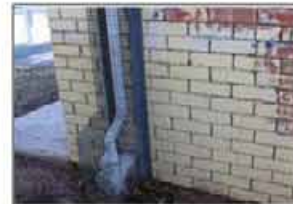
Evidence of graffiti and vandalism
