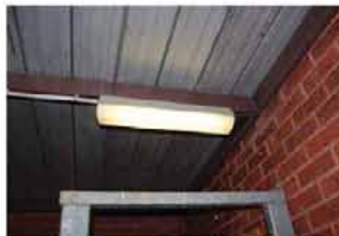
Galvanised finish to ceiling makes building interior dark John McEwen Reserve
