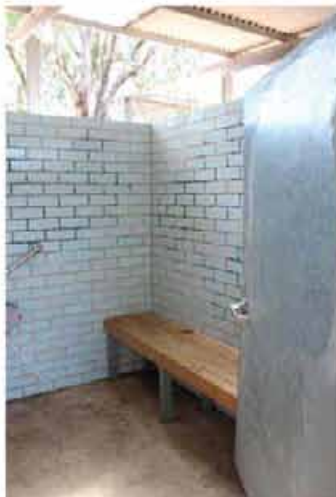
Gap between top of wall and roof increases natural light inside facility. All Abilities Playground, Shepparton
