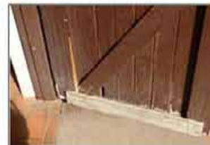
Fixtures and fittings are aged and subject to ongoing maintenance
