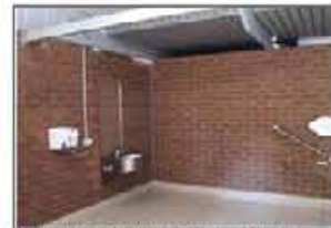
Heavy materials internally, issue with water pooling
