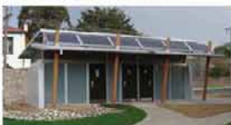
Solar panels on public toilet. Image sourced from the internet.
