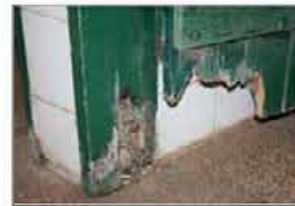
Vandalism and graffiti evident
