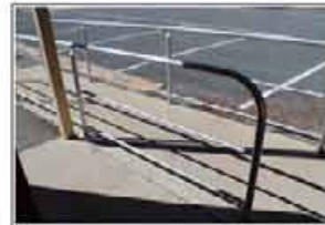
Handrails along entry ramp and tight turning space for wheelchairs
