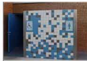
Entrance screens to facilities
