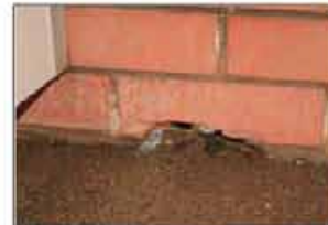
Holes drilled into brick wall to allow water to drain out
