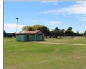
Well defined access to facility, clear sightlines
