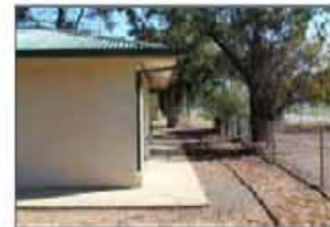
Entrance to the back of site
