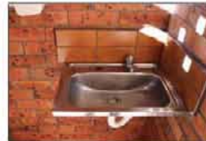
Gaps in the brickwork provide direct sunlight
