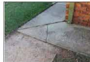
Narrow access path
