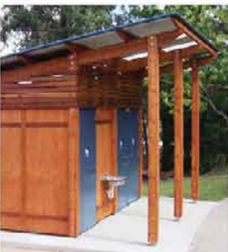
Outside sink protected by roof overhang in this prefabricated public toilet http://www.landmarkpro.com.au
