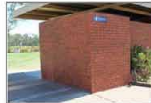
Confusing entrance leading to other side of building
