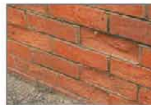
Damage to external bricks, from irrigation system in adjoining park
