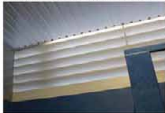
P-Kight painted grills provide natural light and ventilation, but restrict access. Fraser Street, Shepparton
