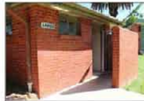
Entrance into facilities obscured by brick wall
