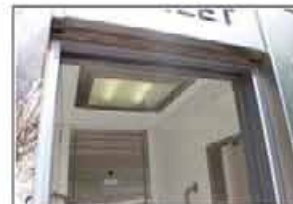
Artificial light only inside facility
