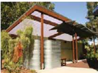
Water collection and reuse, PV cells and recycled materials used at the Eco toilets at Perth Zoo http://www.perthzoo.wa.gov.au
