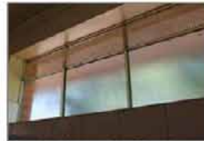
Enclosed windows, restrict ventilation and lighting
