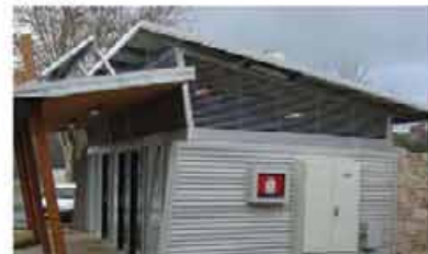
Steel slats provide natural light and ventilation, but restrict access. Image sourced from the internet
