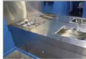
New internal point and renovation works
