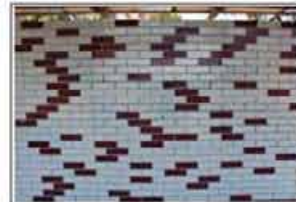
Patterned wall surface
