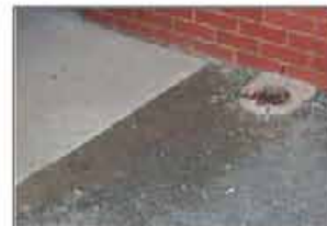
Water pooling at entrance
