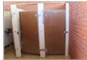
Internal fittings and finishes in poor condition
