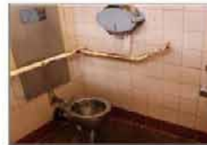
Internal fittings in poor condition
