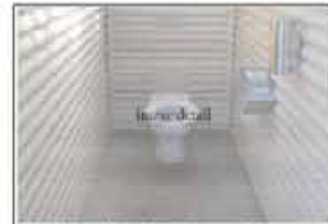
Individual cubicle with good natural light. Corrugated iron difficult to clean/maintain
