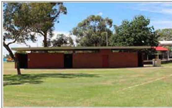
View of facility from Victoria Park Lake. Entrance to the cubicles face the lake.
