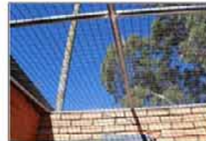
Safety mesh on the roof to restrict access
