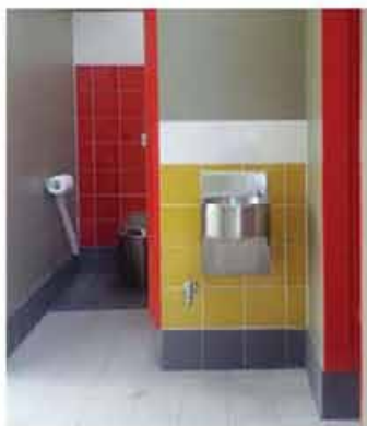
Tiled floor and wall finishes http://www.cocoondesign.com.au
