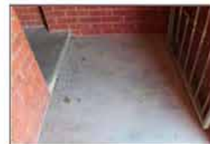
Trip hazard at entrance
