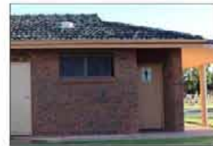
Access into cubicles is recessed and not obvious
