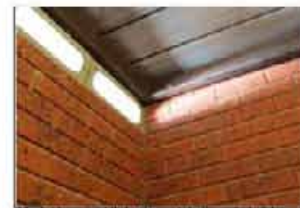
Limited natural light through hollows in bricks and louvers
