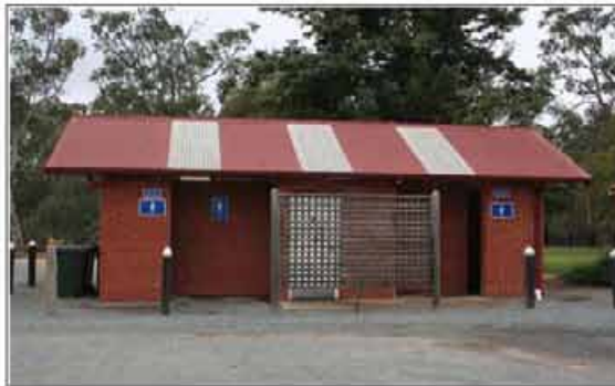
Stand alone building, modesty screen only effective for accessible cubicle
