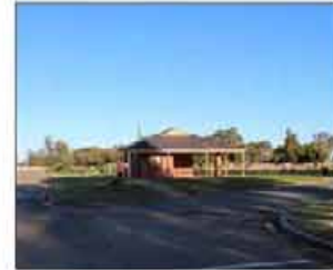
Clear views to facility
