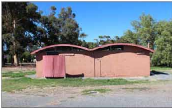
Stand alone facility to the back of site and adjoining primary school
