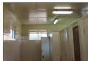
Finishes, fixtures and fittings are aged
