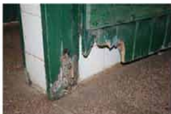
Damaged door Ferruri Park Shepparton
