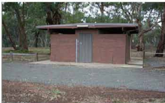
Sound along building between the lake and camping reserve
