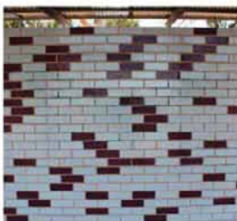
Coloured brick pattern detracts from residual graffiti All Abilities Playground, Shepparton
