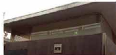
Perspex and perforated steel provide natural light and ventilation, but restrict access. Bendigo
