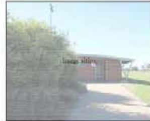
Entrance obscured by vegetation
