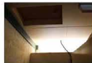
Internal lighting is not adequate
