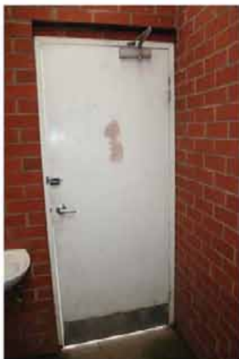
Door damaged and incorrect size Riverbank Gardens, Murchison
