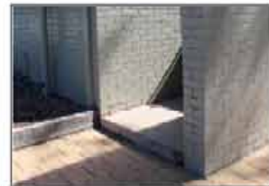
Trip hazard at entrance to building
