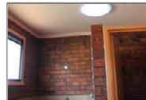
Inadequate internal lighting
