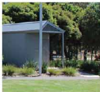
Low planting around toilet block does not restrict views Judd Park, Merrigum
