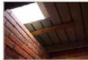
Skylight improves natural light, but internal light is still inadequate
