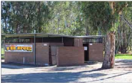
Sound alone building within sports precinct, at back of site adjoining bushland reserve
