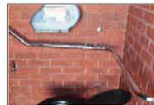
Recent renovations included the replacement of fixtures
