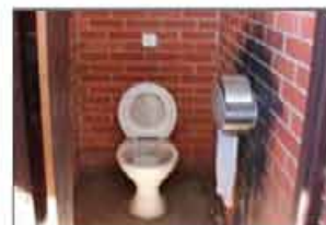
Evidence of vandalism
