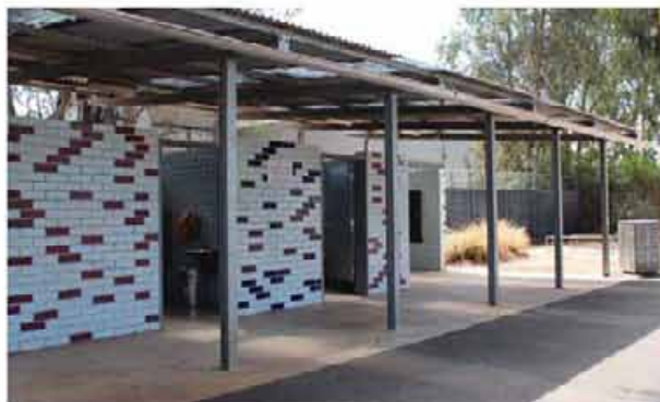
Large opening between top of wall and roof allows excellent natural light and ventilation. All Abilities Playground, Shepparton
