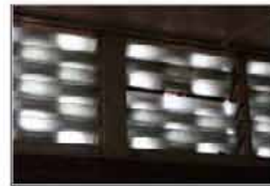
Louvers and hollow bricks restrict natural light
