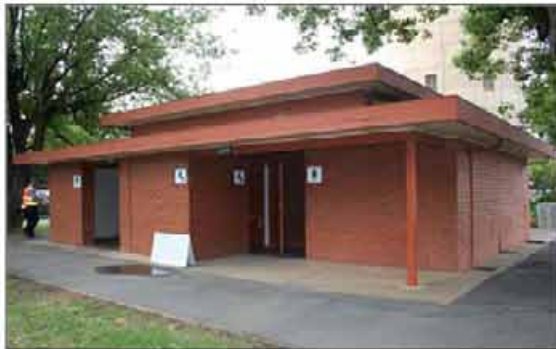
Defined pathways around facility, damage to path from tree roots.
