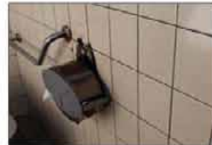
Evidence of vandalism and graffiti
