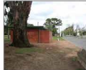
Adjoining car park and Highway
