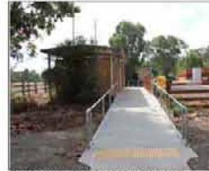
Ramp access with TGS and handrails from activity areas
