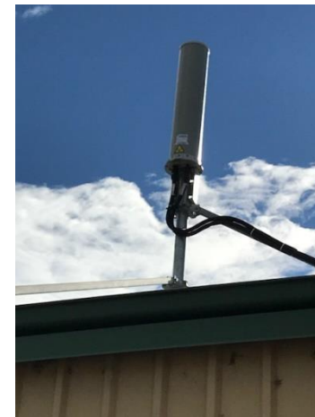
Telstra antenna installed in 2018 to help alleviate mobile reception issues.
