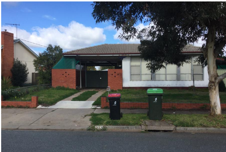
View of 24 Kennedy Road
