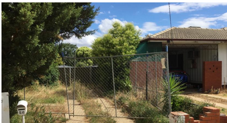
View of existing driveway and dwelling to the west of the land
