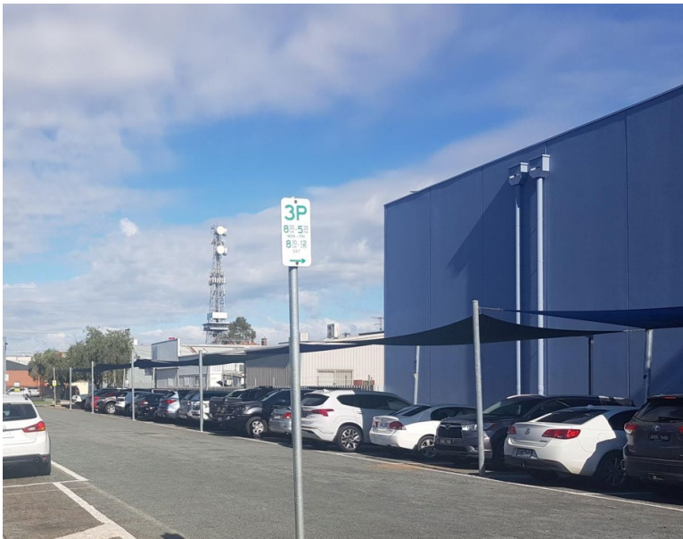
Figure 13: View West of rear side of 92 Nixon Street
