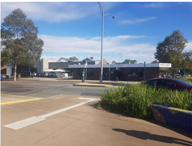
Figure 12: View West of 115-121 Maude Street
