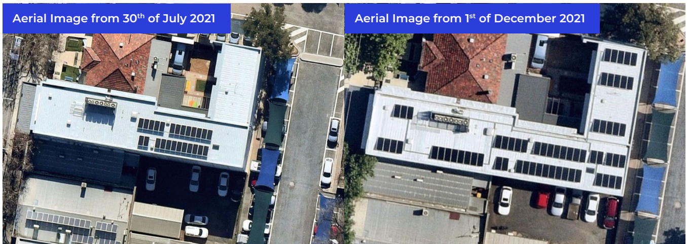
Figure 29: Aerial Images of 123-129 Maude Street showing additional solar panels
