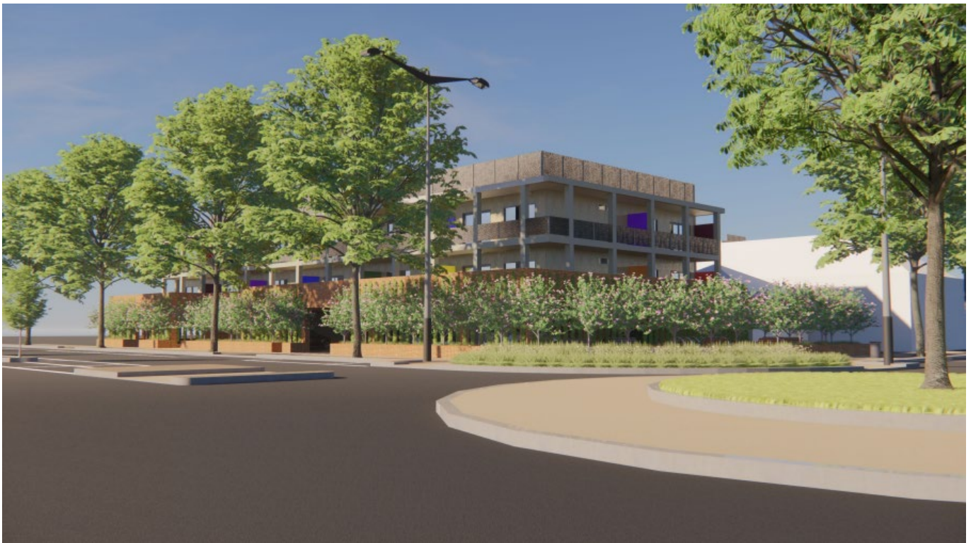
Figure 16 View of proposed development from the corner of Maude and Nixon Street
