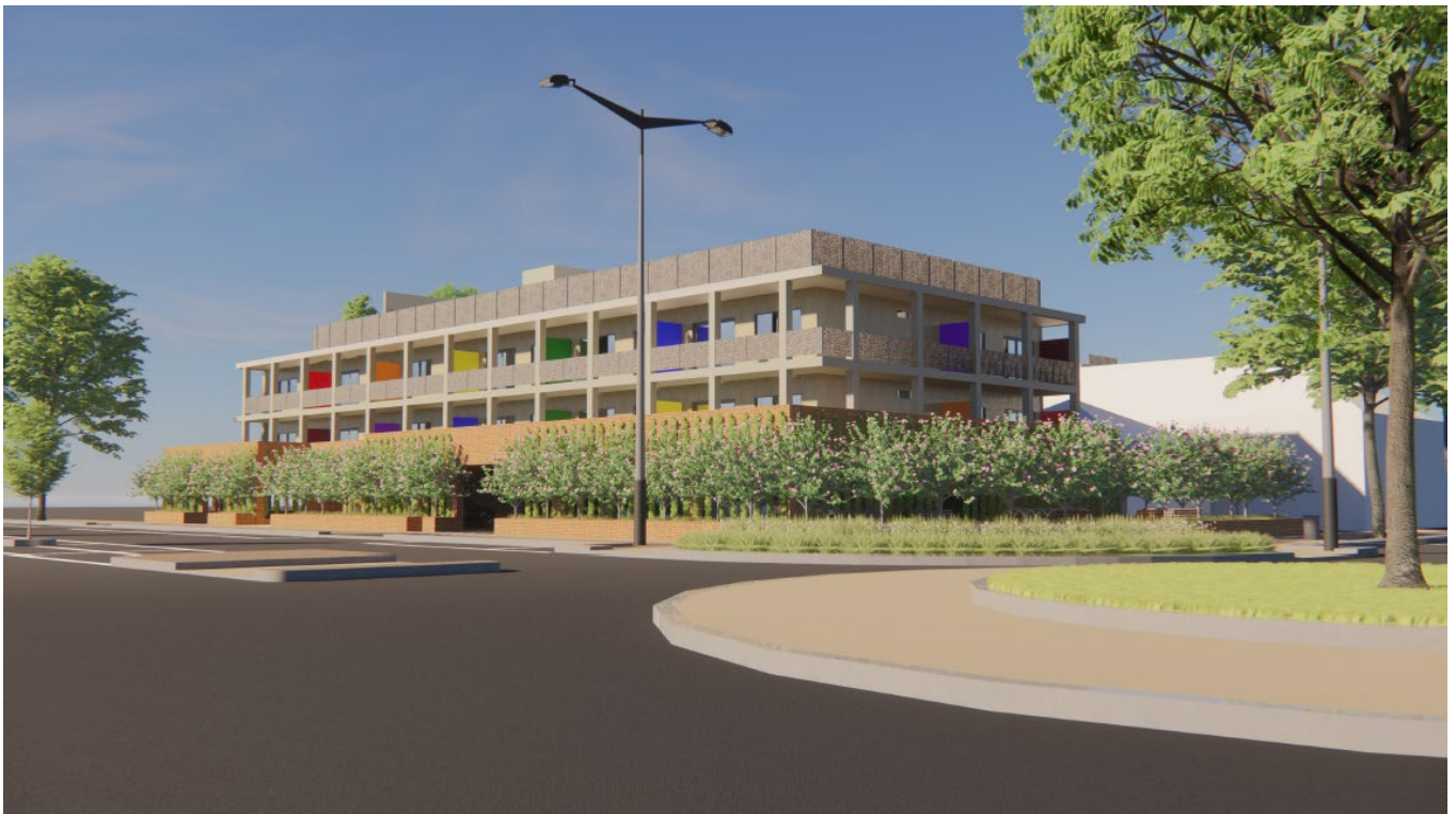
Figure 31: Proposed Concept Design Response, Corner View with Existing Trees to Maude and Nixon Street –
