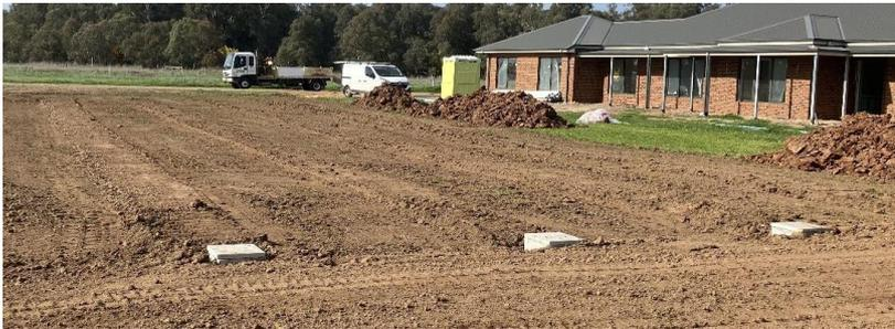
Image 16: Completed work – top of each trench is domed above natural ground so that surface water/rain does not sit on top of the trenches.
