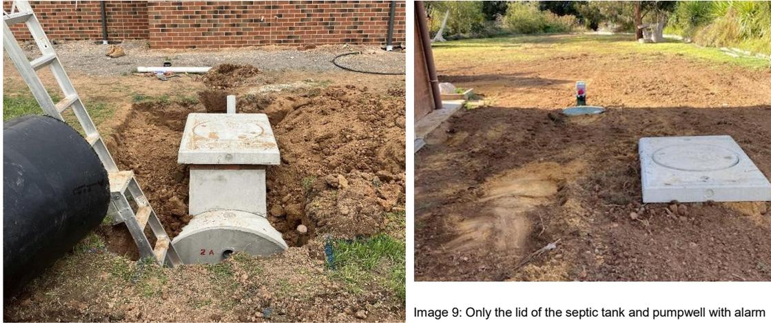
Image 9: Only the lid of the septic tank and pumpwell with alarm are visible when backfilled.
