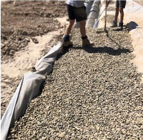
Image 18: Backfilling of Wick Trenches, with Geotextile fabric lining the trench before backfilling with suitable sized rock and arch drain.
