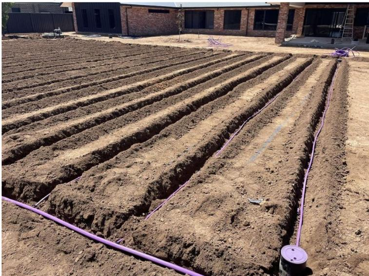
Image 19: pressurized sub-surface drip irrigation
