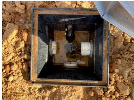
Image 14: Inside the distribution pit installed at the beginning of each trench.
