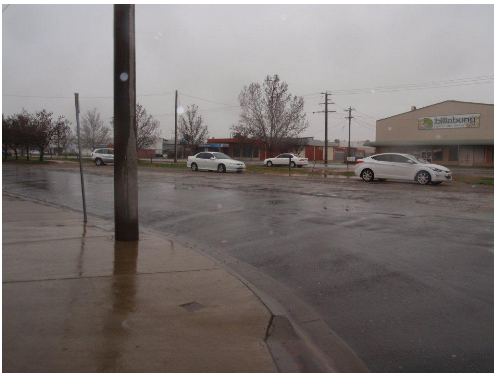
View from milk bar corner of Ash Street and informal parking on south side of Ash Street
