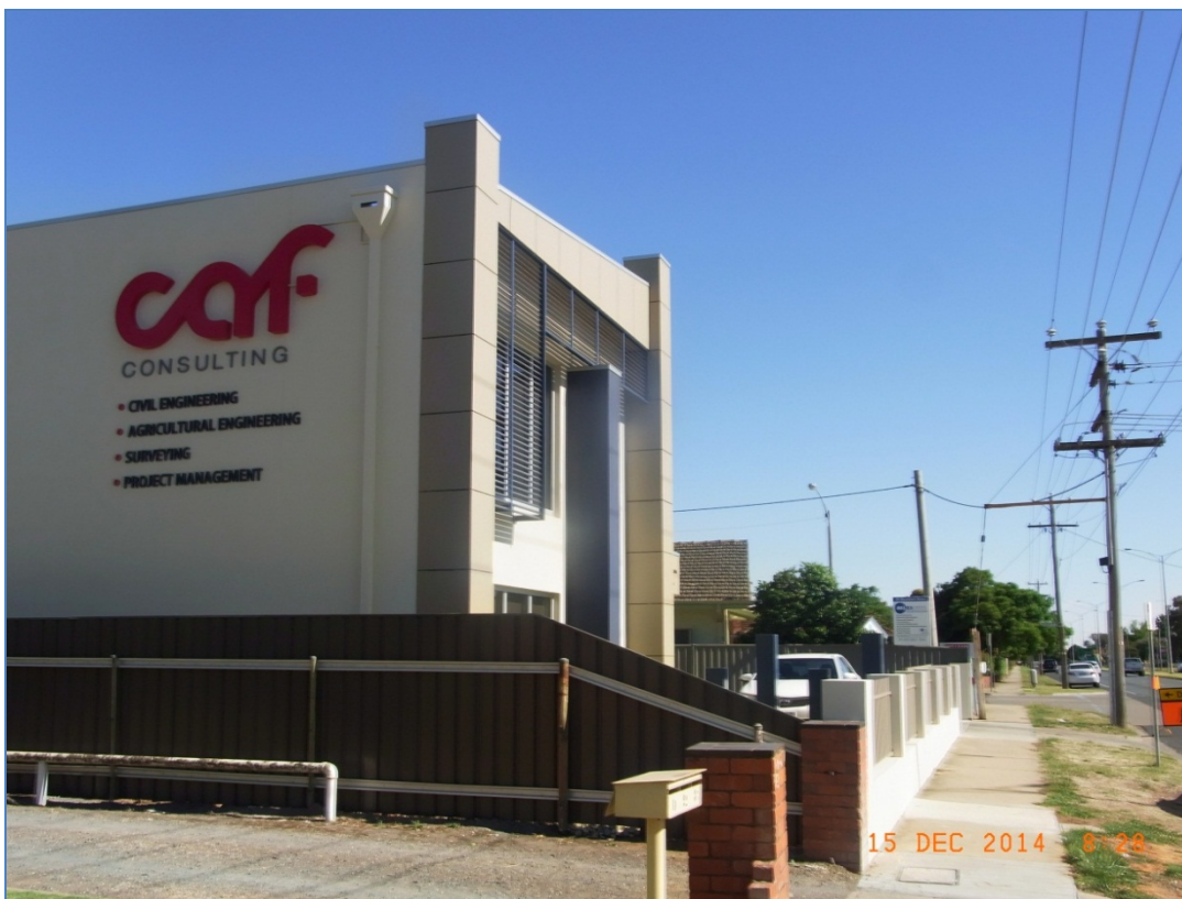
Looking east along Wyndham Street.
