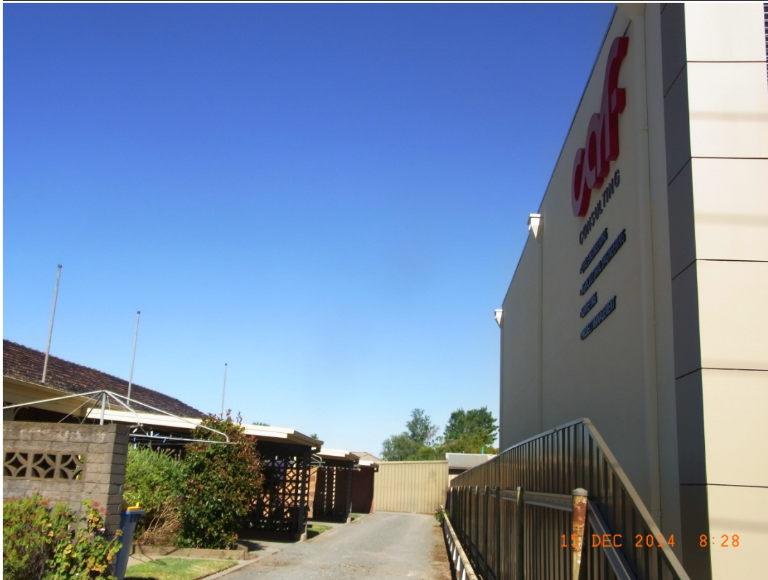
Looking east along the boundary between 38 and 42 Wyndham Street.
