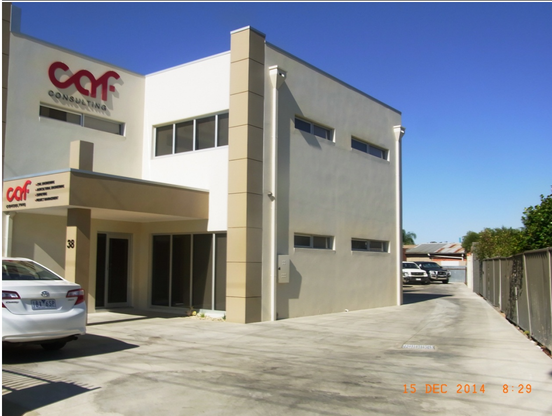
Looking south-west along the boundary between 36 and 38 Wyndham Street.
