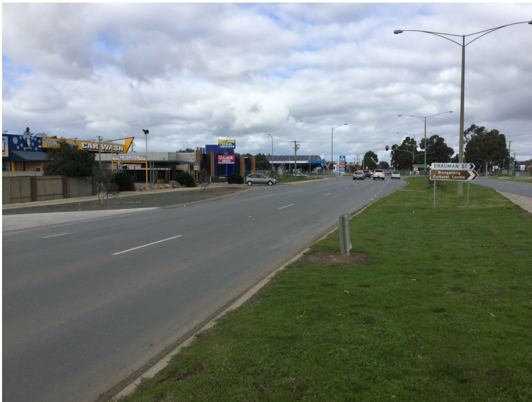
View of Numurkah Road looking south
