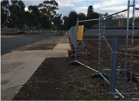
Footpath in Echuca Road looking north
