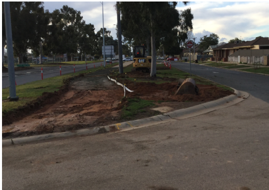
Shared path under construction in the Echuca Road outer separator
