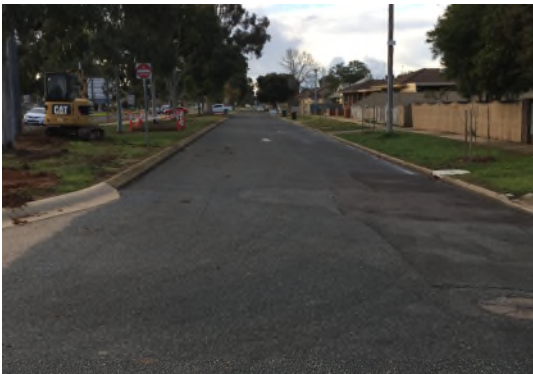
Echuca Road service road looking north
