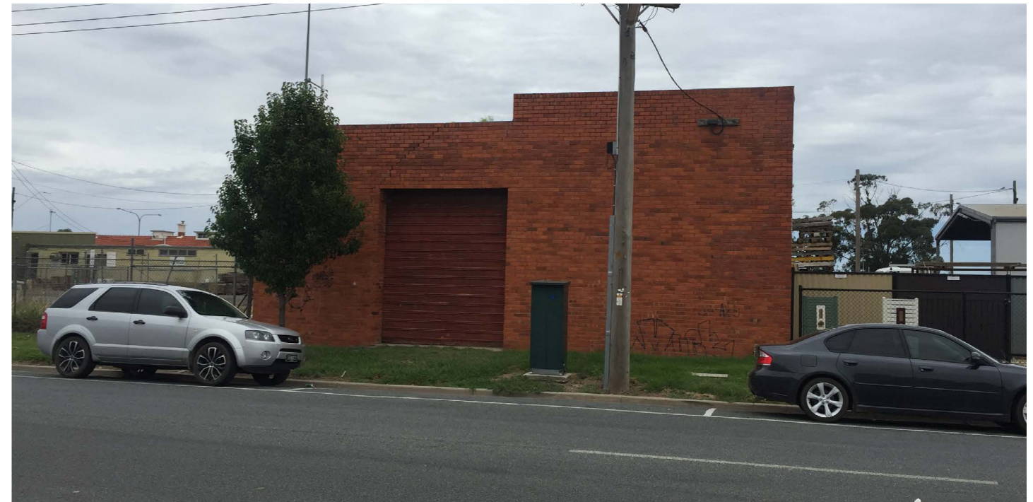
Figure 8 Building No.7 Brick building on Hoskin Street
