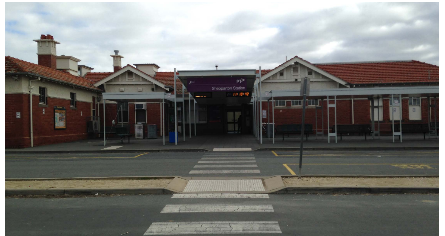
Shepparton Railway Station Entrance
