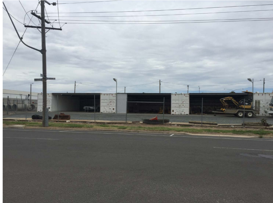
Figure 11 Building No.11 V/Line main Works Depot on Hoskin Street (opposite Rowe Street)
