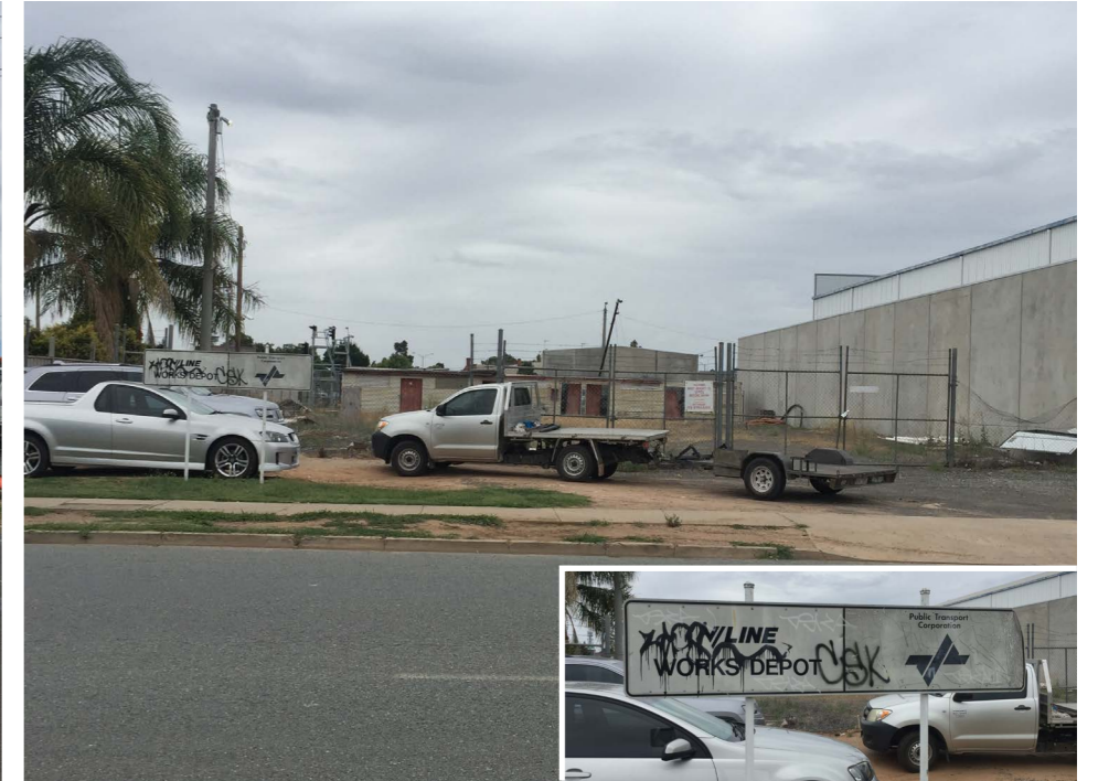
Figure 12 Building No.16 V/Line secondary Works Depot off Purcell Street
