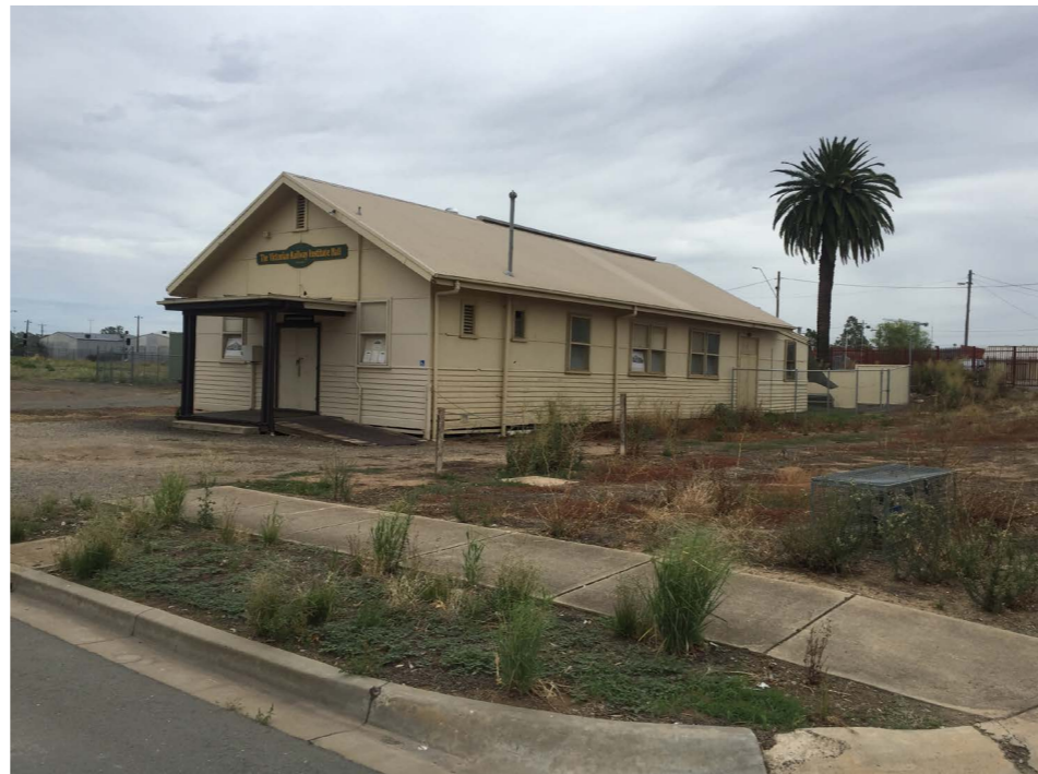
Figure 14 Building No.19 The Victorian Railway Institute Hall
