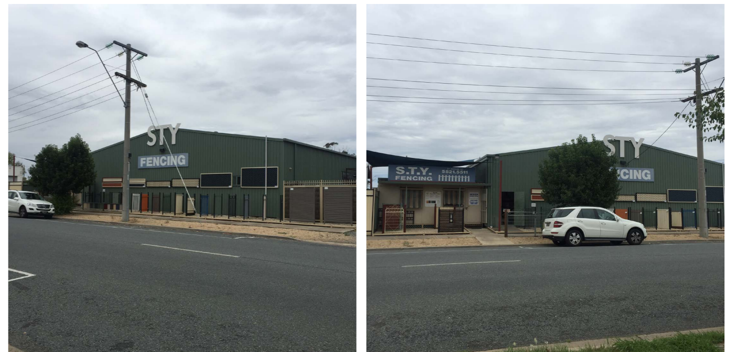
Figure 7 Building No.6 Sty Fencing warehouse and yard on Hoskin Street
