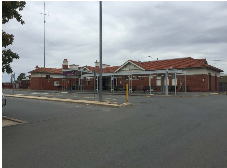
Figure 13 Building No.18 c1910 Heritage-listed Shepparton Railway Station
