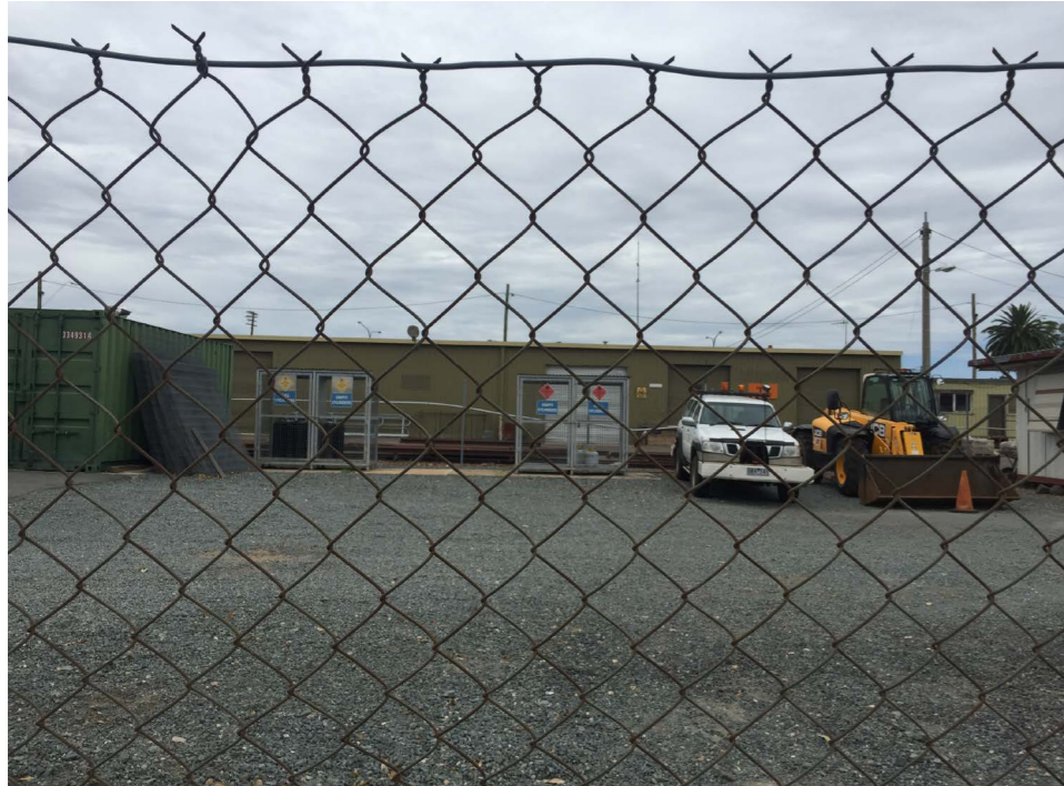
Figure 10 Building No.10 V/Line green storage shed behind Works Depot (opposite station platform)
