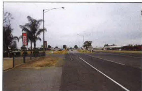
Figure 9: Goulburn Valley Highway view South
