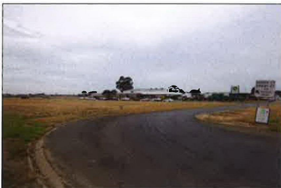
Figure 5: Subject Site viewed from Goulburn Valley Highway
