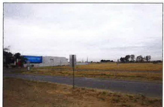
Figure 6: Subject Site viewed from Goulburn Valley Highway
