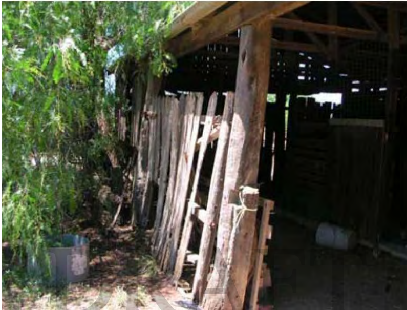
Stable building 1- This structure has been constructed using a variety of building techniques and materials. The structure is eclectic and cobbled together in a relatively ad hoc manner.
