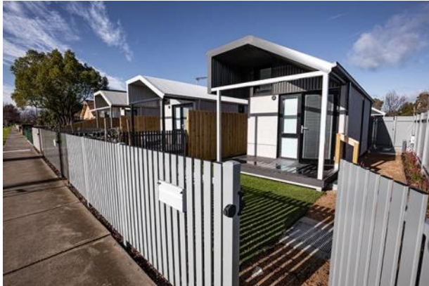
Figure 6: Harris Transportable Housing, Melbourne
