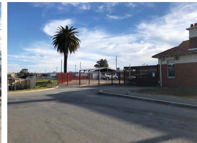
4. Close-up view from Station Drop Off Area
