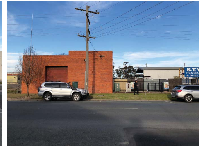
2. Close-up view from Vaughan St West - Existing brick building to be demolished for new entry to pedestrian overpass
