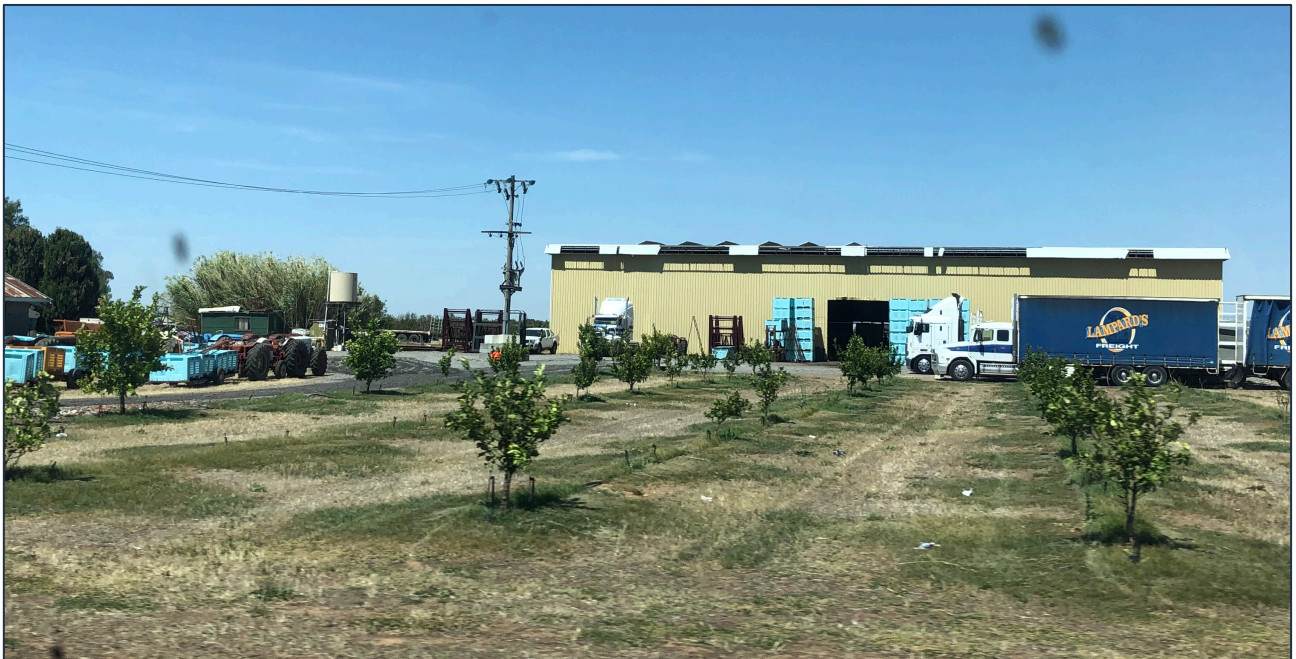
Coolstore and packing sheds (RMCG)
