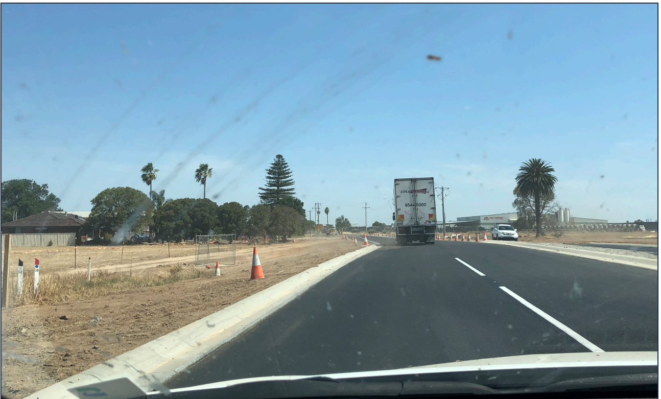
Upgrade of Doyles Road (RMCG)
