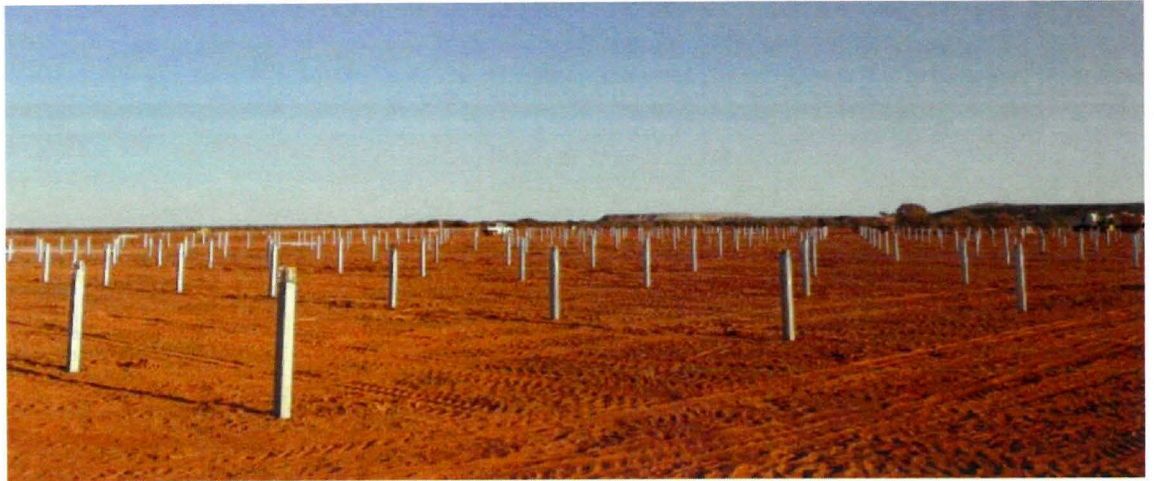
Figure 4 Example of mounting poles driven on previous project in Western Australia
