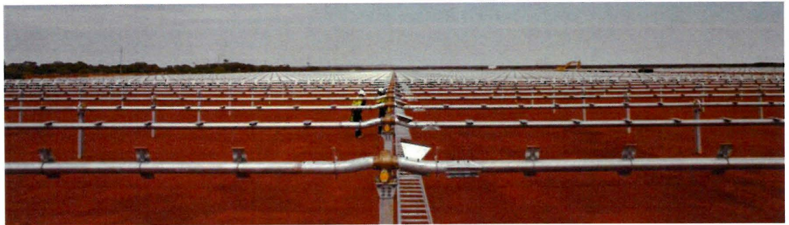
Figure 5 Example of single-axis mounting system before panel installation
