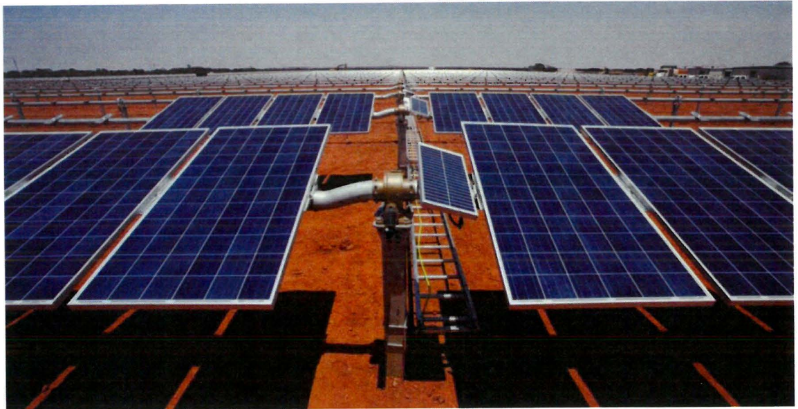
Figure 6 Example of single-axis mounting system after panel installation
